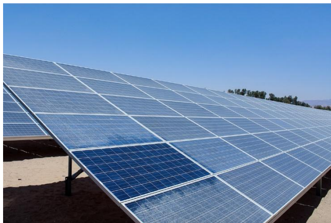
Fig. 2. Array of solar panels accumulated by dust.
